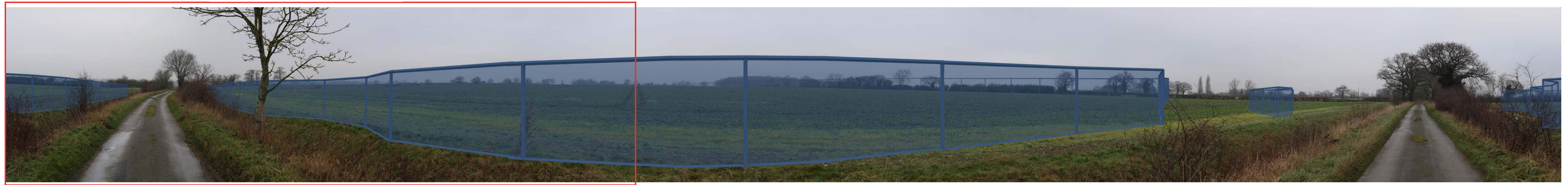
Site Context Photograph (1 of 2)
